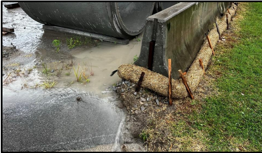
Straw waddle installation near outfall 002
