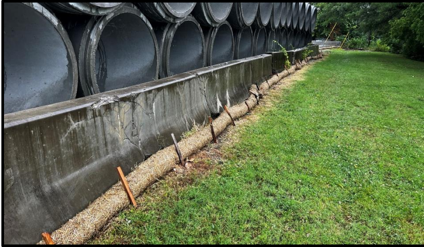
Straw waddle installation near outfall 002
