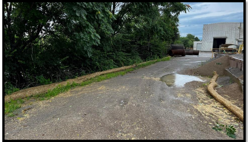
Straw waddle installation near outfall 003
