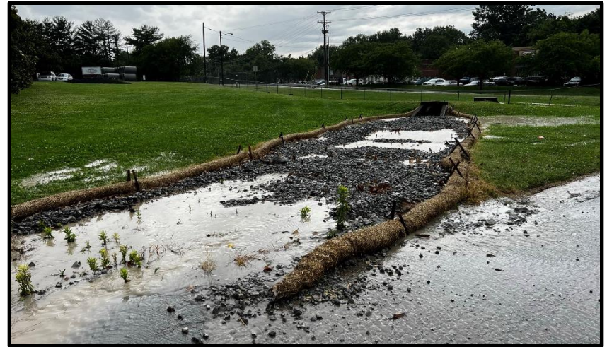
Straw waddle installation near outfall 001
