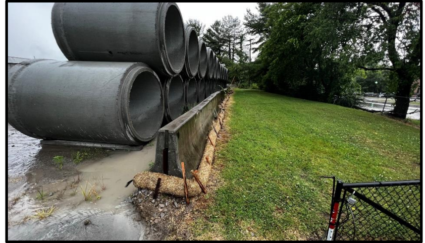
Straw waddle installation near outfall 002
