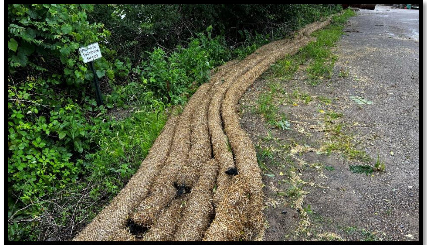
Straw waddle installation near outfall 003
