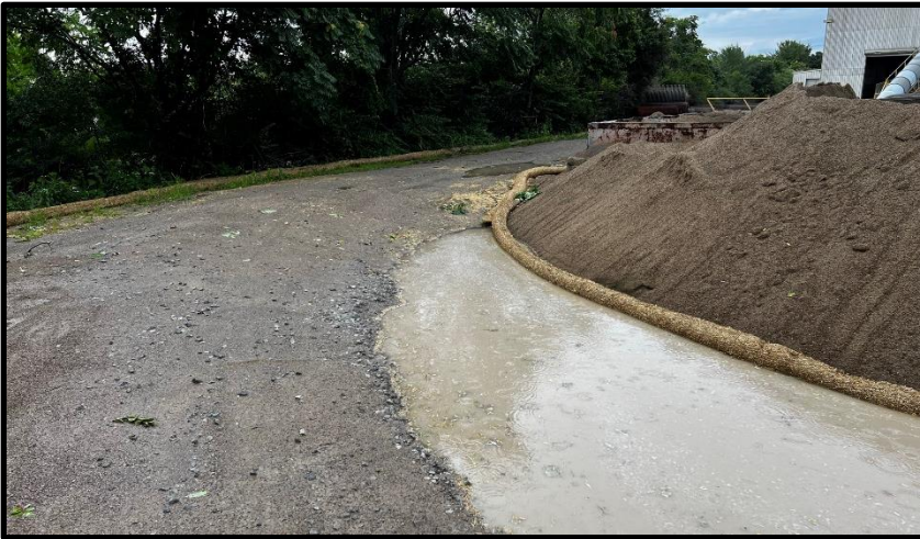
Straw waddle installation near outfall 003
