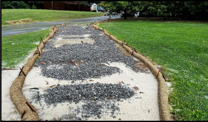
Straw waddle installation near outfall 001
