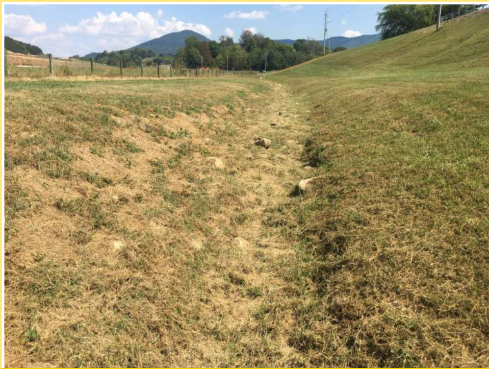
Photo 1 – General view of Clear Creek facing upstream of existing culvert inlet.
