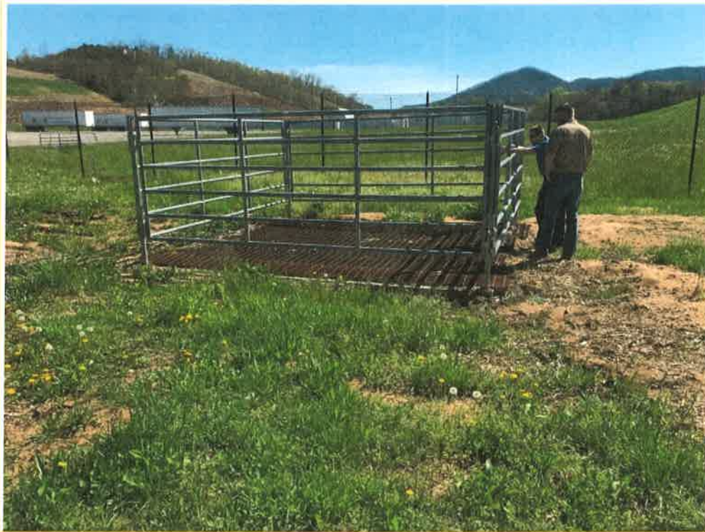
Photo 11 – Existing, grated junction box and begin impact proposed location.
