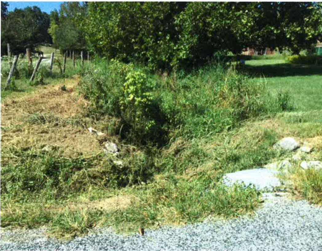
Creek Crossing #9 – trib. of Sheppard Branch
