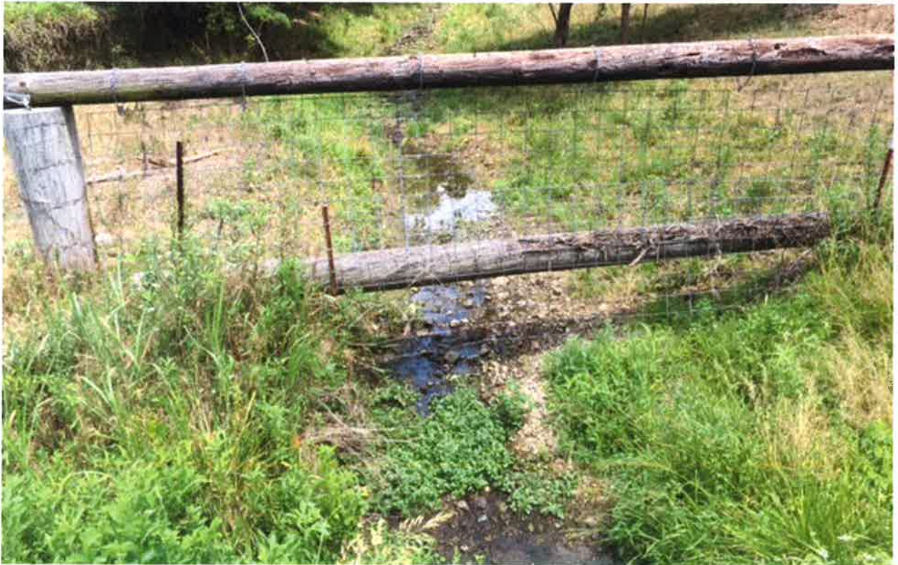
Creek Crossing 2 – Unnamed Tributary to Richland Creek, Looking North
