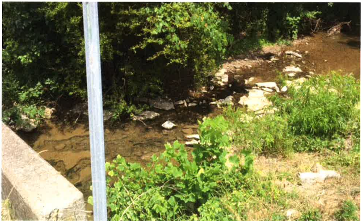
Creek Crossing 3 – Troy Fork Creek, Tributary to Richland Creek, Looking North West
