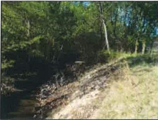
Figure 53: Slope repair using grouted Rip-rap; note the cantilevered pipe in the background
