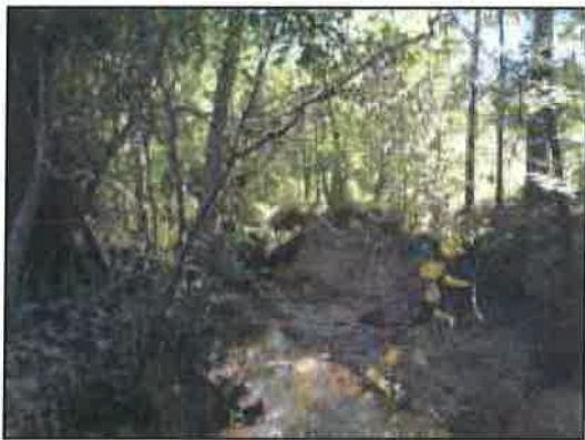
Figure 42: Looking downstream at bank Erosion shown in figures 40 and 42
