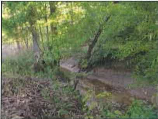
Figure 34: View from edge of the washout noted in figure 33; note the root ball beginning to slide down the slope
