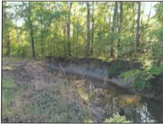
Figure 15: Looking downstream at the disturbed slope
