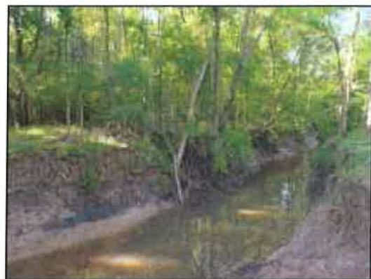
Figure 20: Looking upstream from the end of the failing section of the west bank
