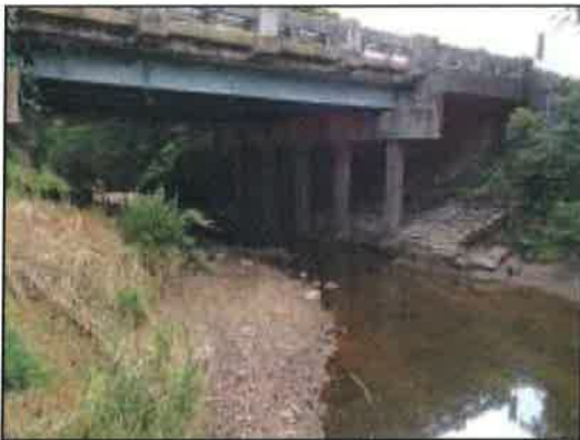
Figure 74: Bridge pilings in 2013
