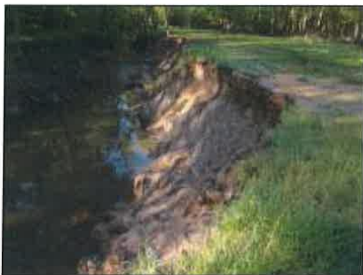
Figure 19: Face of recent bank failure just upstream of the shear crack
