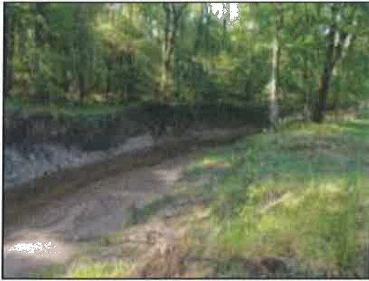
Figure 24: Mid-point of bend with deposits on the inside of the bend; note the bank has laid back on an approximation of a 2:1 slope
