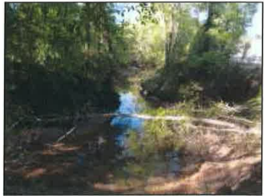
Figure 45: Looking upstream from same vantage point as figure 44; note the short meander pattern and the slope failure of the west bank on the outside bend
