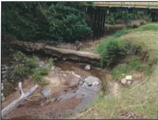
Figure 72: Water line crossing in 2013
