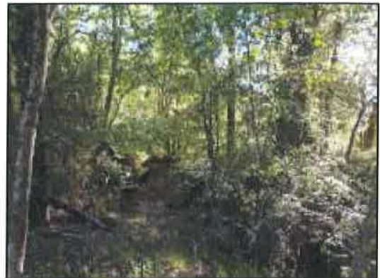
Figure 47: Upper end of the meandering pattern shown in figure 45 looking downstream; note the outside bend erosion in the background
