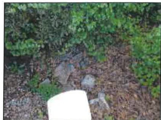
Figure 49: Close up of end of culvert
