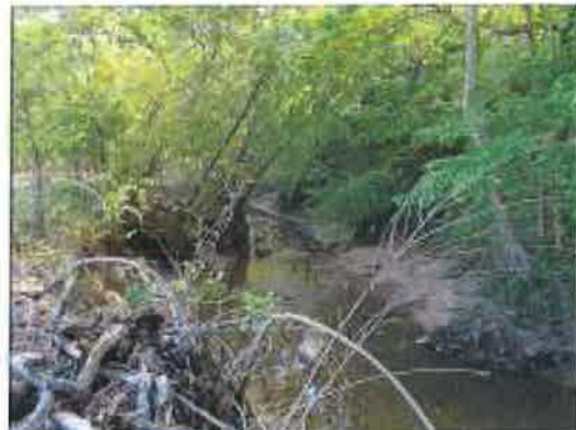
Figure 35: Standing at the edge of bank just upstream of the washout looking downstream
