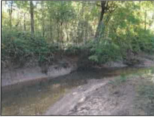
Figure 8: Lower end of next bend; note the deposition on the inside (west side) and the undermining of the east bank
