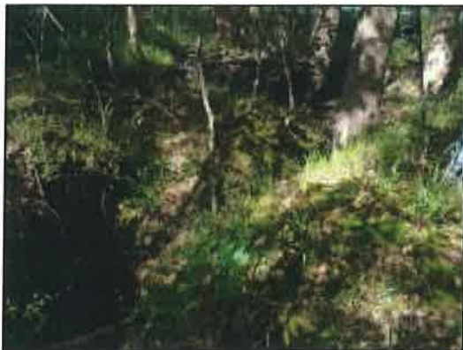
Figure 63: Crevice isolating an area on the west bank
