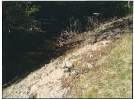
Figure 54: Close up of grouted rip-rap
