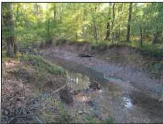
Figure 13: Looking downstream from approximately the mid-point of the bend; the change where the soil profile changes for the upper silty loam to the underlying clay is clearly evident (denoted by black arrow)
