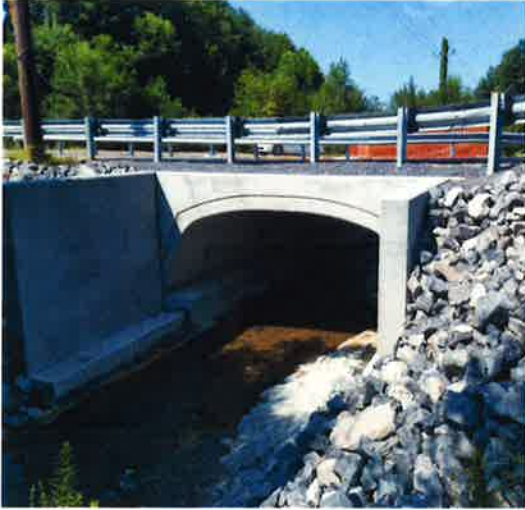
Bloomington Drive culvert replacement
