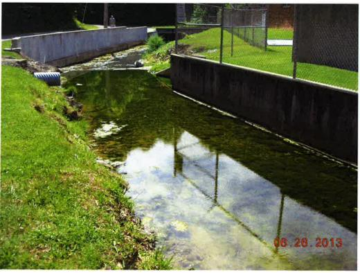
These are photos showing the outtall and just downstream. The heavy algae growth continues here due to both the permitted discharge and the manhole overflow. The system is an sequencing batch reactor (SBR), so the discharge is not continuous. The periodic discharges are released and flush downstream in a slug, then the stream flow returns to the normal low levels.
