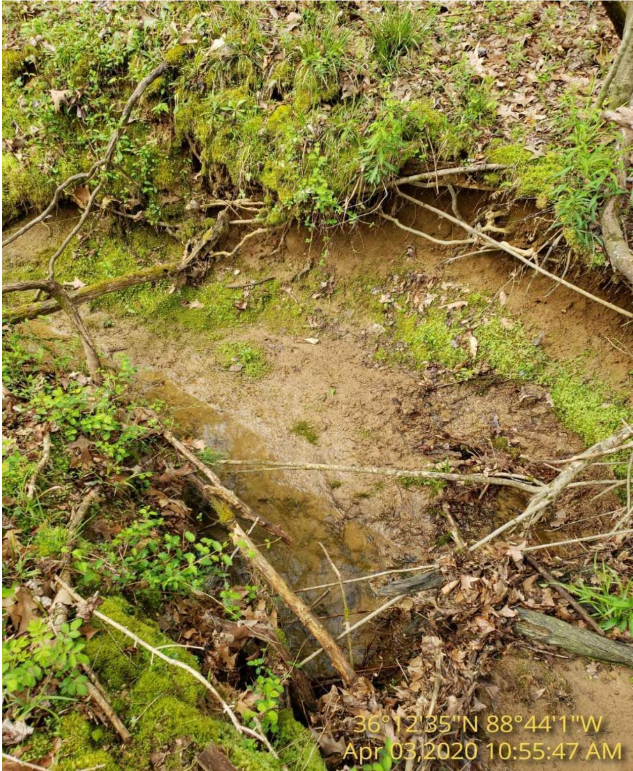
PHOTO 11: View of a small grade control as we continue south. Stream.
