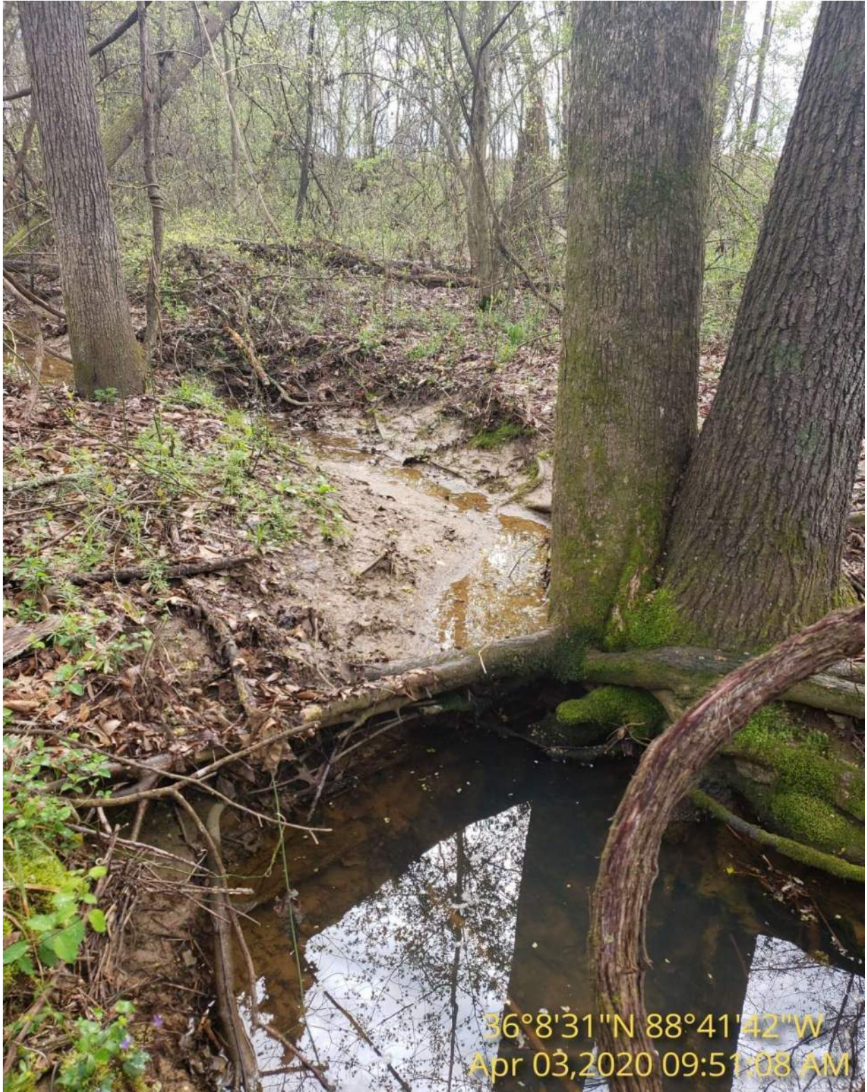
PHOTO 12: View of a large grade control and a deep pool of water.
