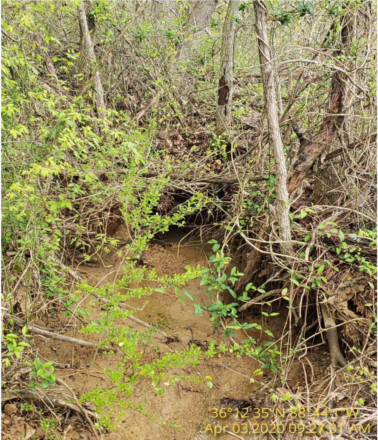
PHOTO 2: View of the channel looking east, showing a large grade control.
