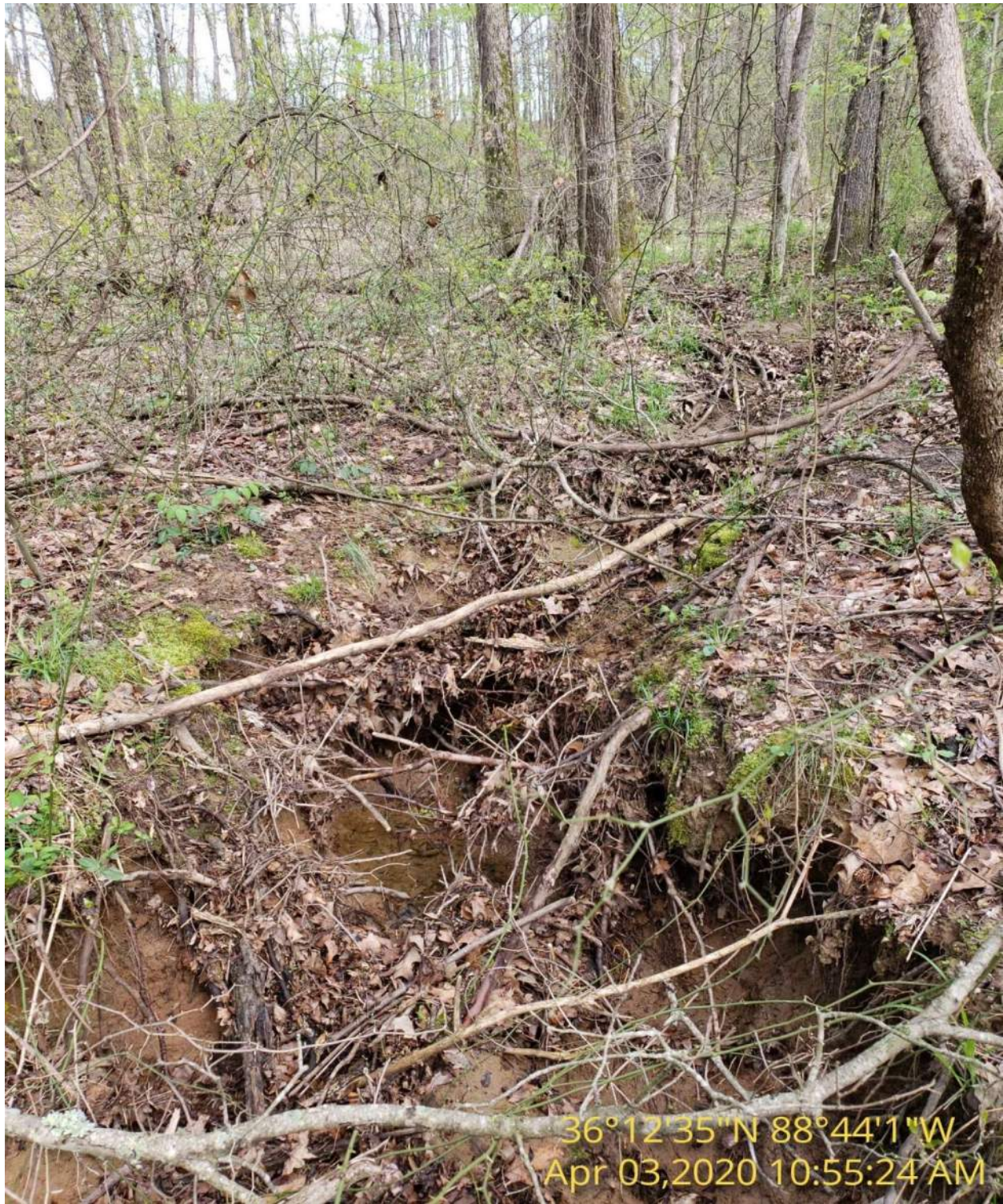
PHOTO 10: View of channel looking north at a large headcut. Stream.
