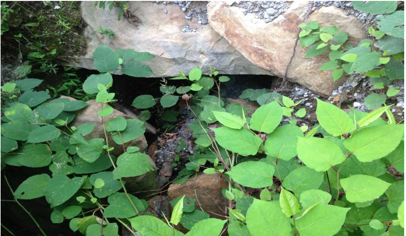
Stream 9 lower culvert
