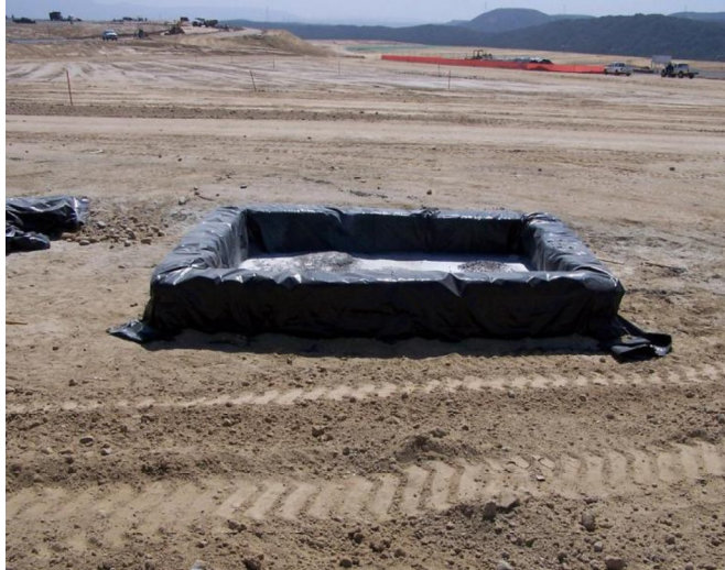
CONCRETE WASHOUT
