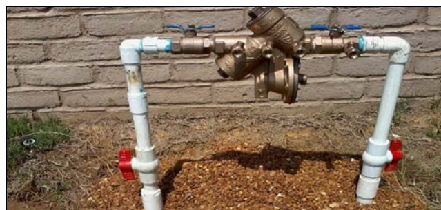
Example Installation of Irrigation Backflow Preventer
