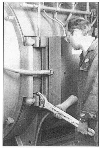
Figure 8-36: Tighten Hinge Bolts
