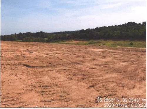
Photo 1. View northeast over the rea with new cover. Note the erosion rills in the bare soil.
