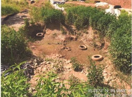
Photo 7. Liquids flowing from under the phase IV liner into the temporary sump.
