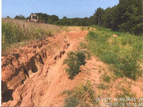
Photo 5. Erosion in the run-off ditch at the northwest corner of phase III.
