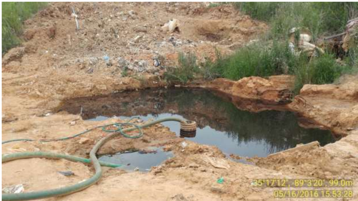
Picture 3. Primary dewatering area on the Phase III liner. This is in the area near where the original Phase IV leachate collection pipe attempted to tie-in to the Phase III leachate system. The indentation in the ground on the middle left of the picture is where this area flows into a second pit dug by Hardeman County Landfill's construction contractor, Ronald Franks Construction.
