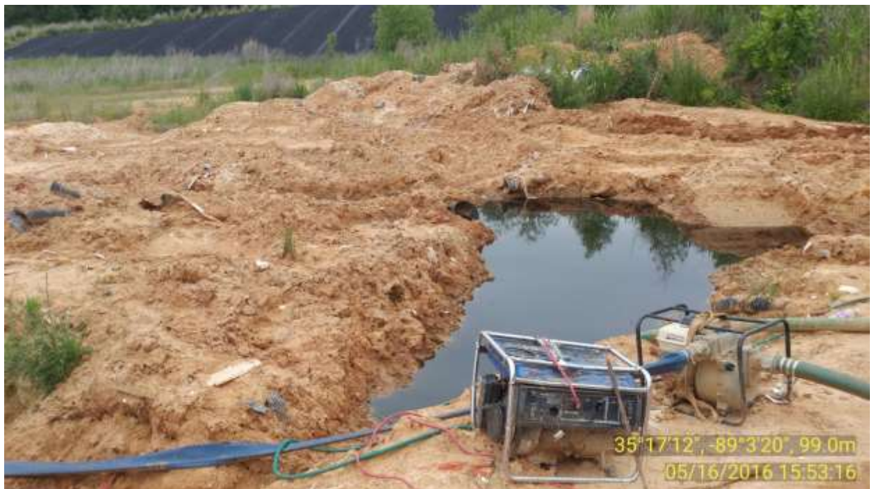
Picture 4. View of the "secondary containment" pit which appears to be located on both the Phase III and Phase IV liners. Two 3-inch pumps which were used to dewater the work area are pictured in the foreground.
