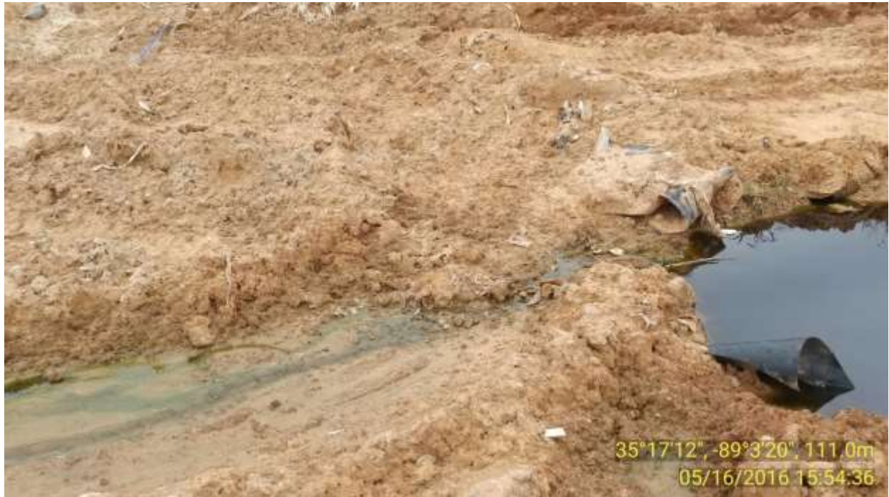
Picture 5. Leachate flowing out of the “secondary containment” area into an excavated channel on the Phase IV liner.
