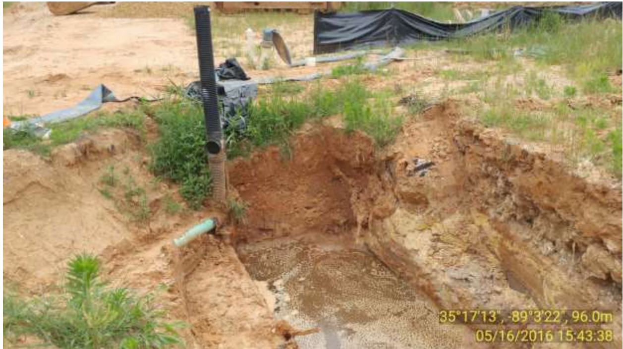
Picture 1. Stack where temporary leachate by-pass (green-blue colored pipe) joins with leachate line to run towards the leachate collection tank.
