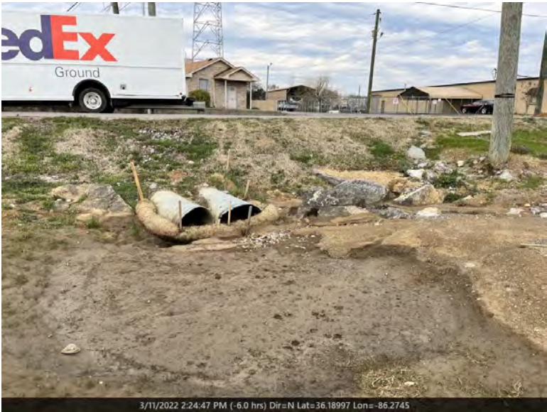
11 Additional view of WWC-2/UDF-2 south of Briskin Lane at silt-filled culvert, facing downstream/north. Silt was beginning to crack because of dry conditions.
