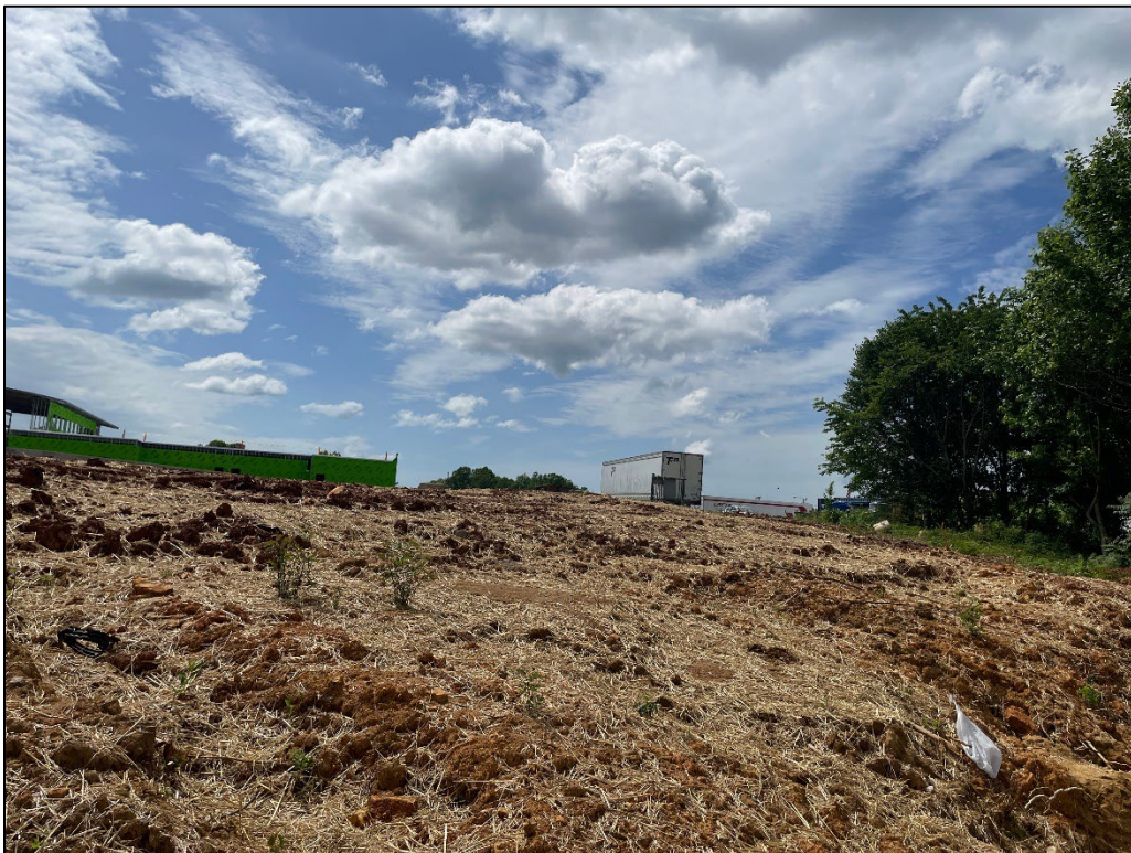
Picture 4. Photograph of fill material to the north of the identified wetland area (WET-A). This area has been seeded and strawed and would be up-gradient from the proposed riprap slopes.
