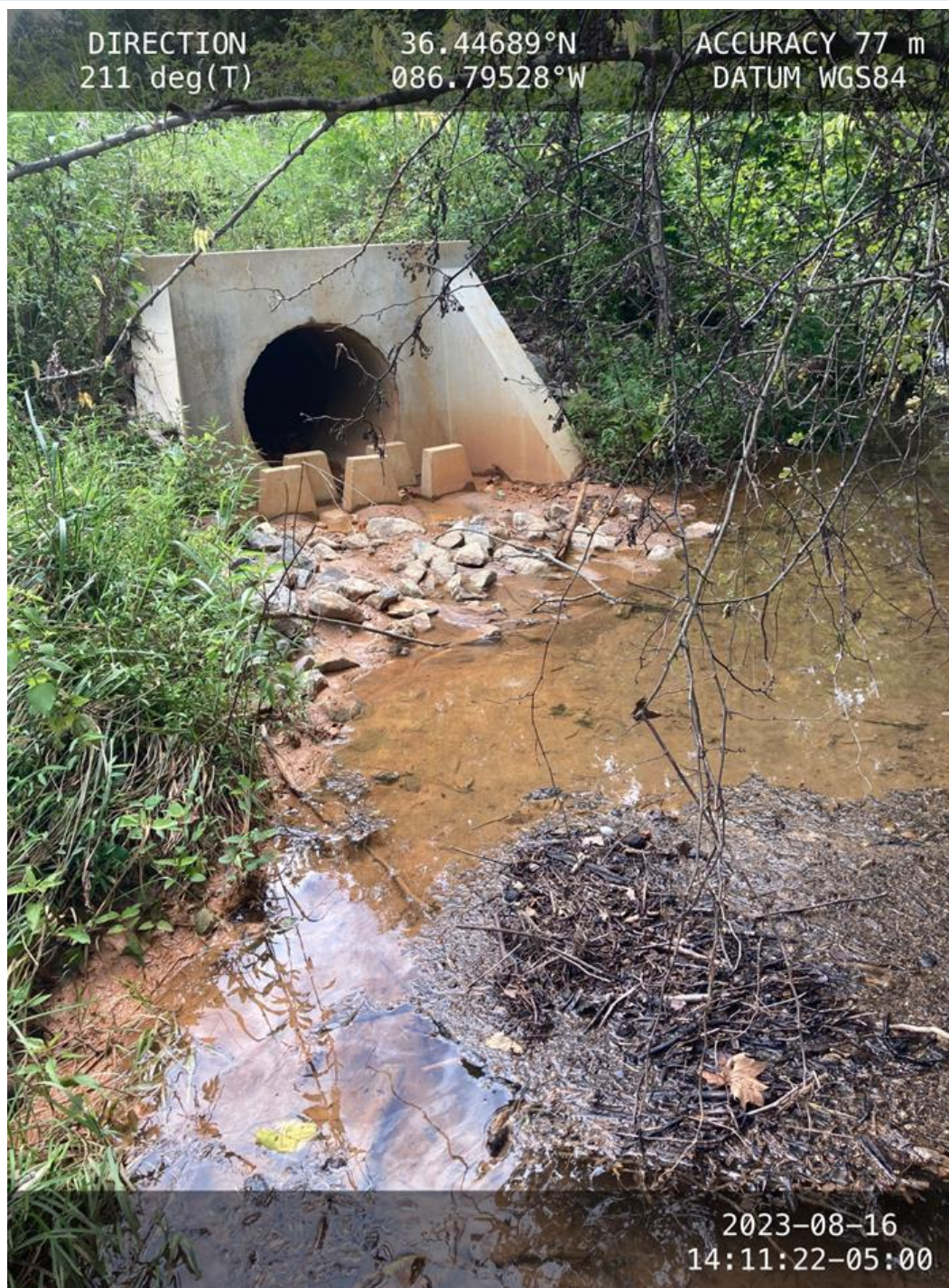
Attachment 2: sedimentation of unnamed tributary to Long Branch at outfall located below failed sediment basin
