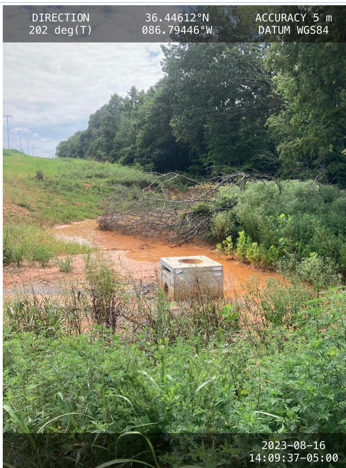
Attachment 1: View of failed sediment basin in need of maintenance.
