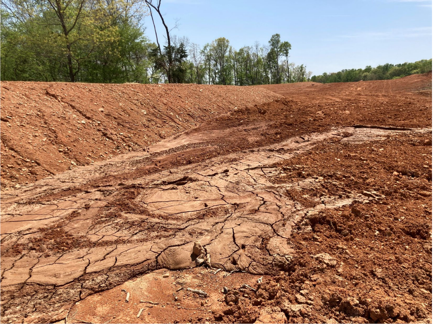
Photo 3: Area of potential conduit to spring and pond below Yellow Creek Quarry. Stormwater drainage from disturbed area pools here behind the berm and slowly infiltrates through the berm or potentially into the spring. The facility needs to redirect this drainage into the mine pit or sediment basin, stabilize the disturbed area that they are not immediately expanding into, and protect this area with BMPs to prevent sediment laden water from draining into this potential conduit.
