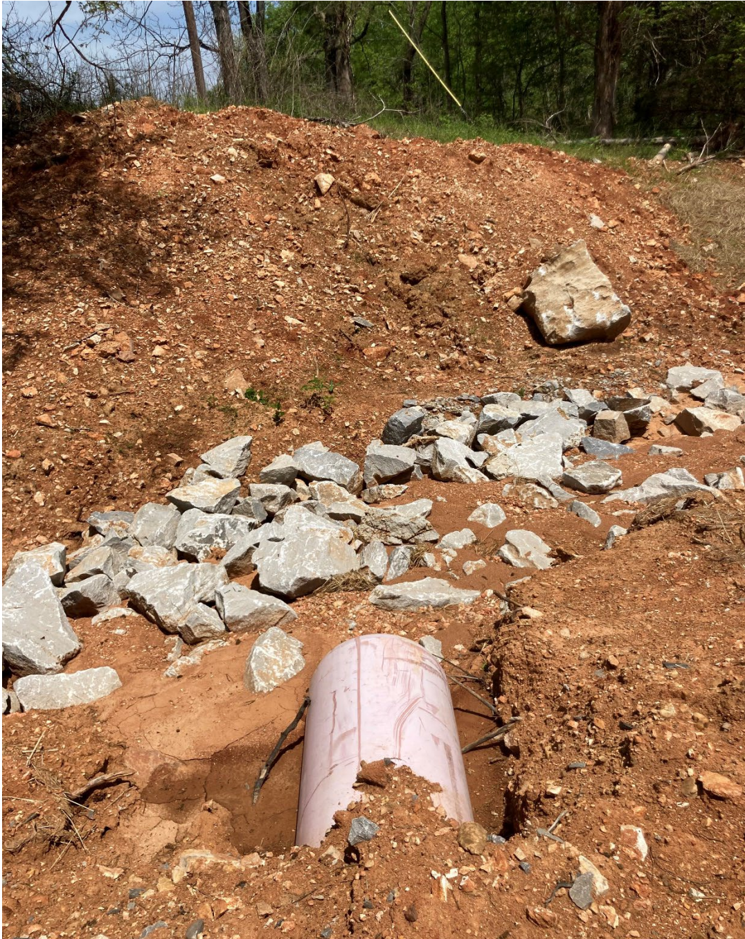
Photo 10: Large amounts of unstabilized soil at culvert at upper portion of driveway.
