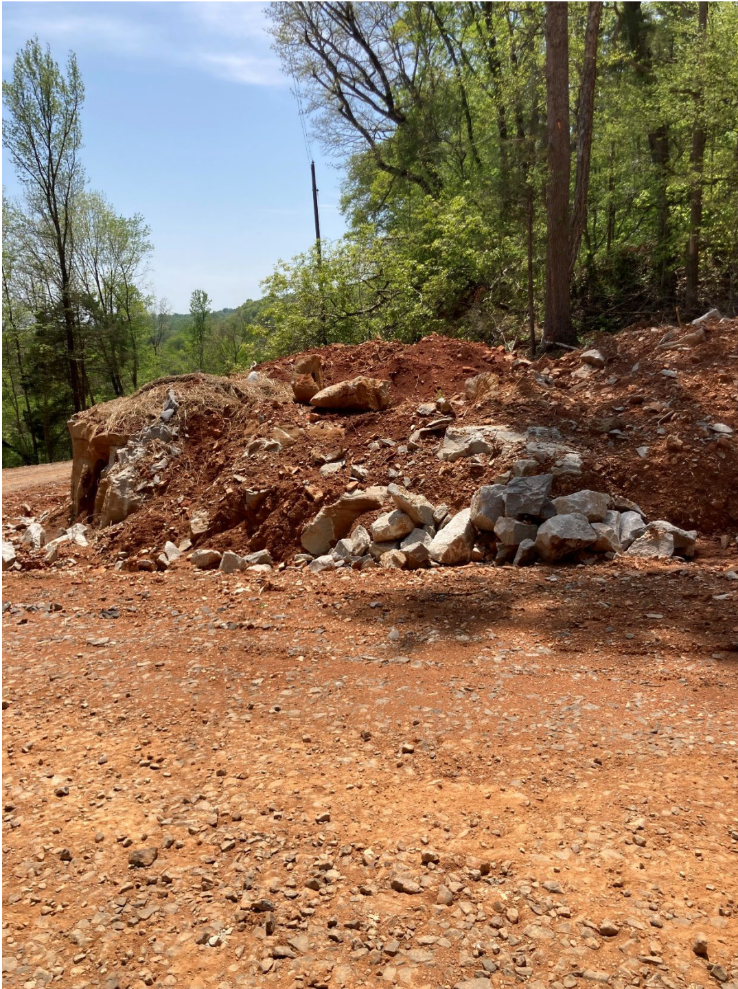
Photo 9: Large amounts of unstabilized soil at the upper portion of the driveway.
