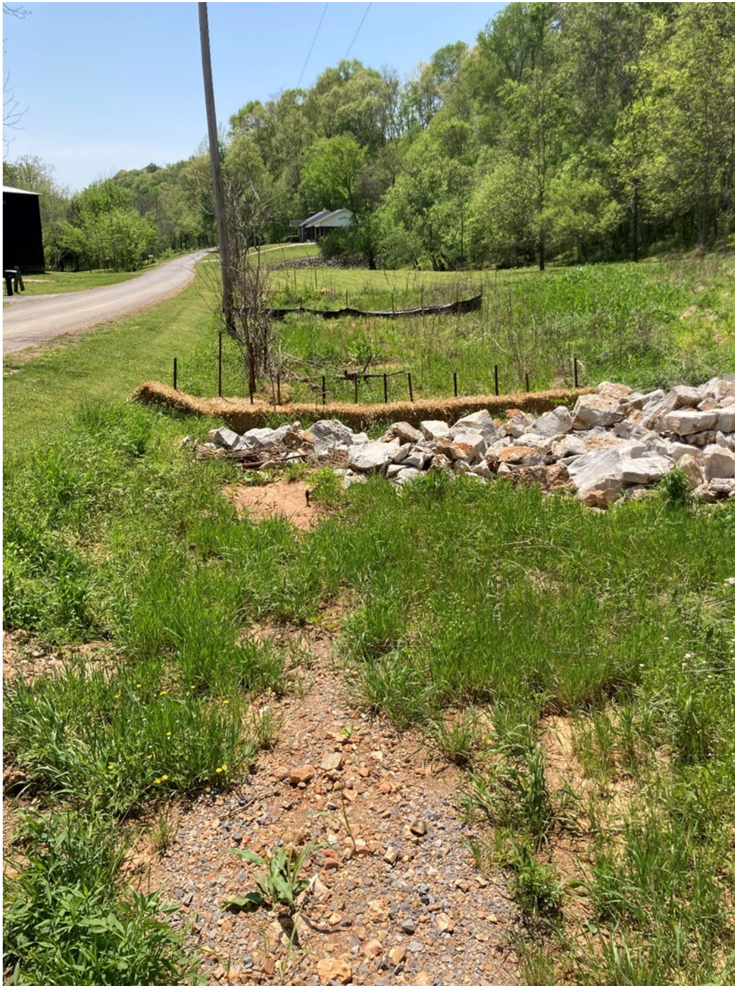
Photo 6: Series of BMPs at the facility entrance to treat stormwater before it leaves the site.
