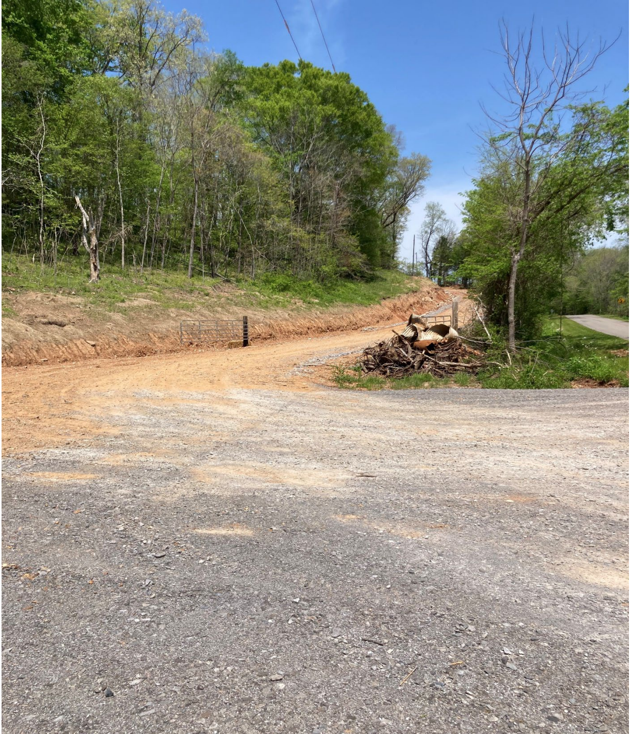
Photo 4: Tracking pad at the entrance of the facility.
