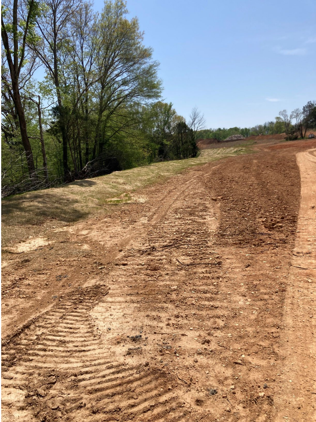
Photo 14: Photo of stabilized berms at the edge of the disturbed area.
