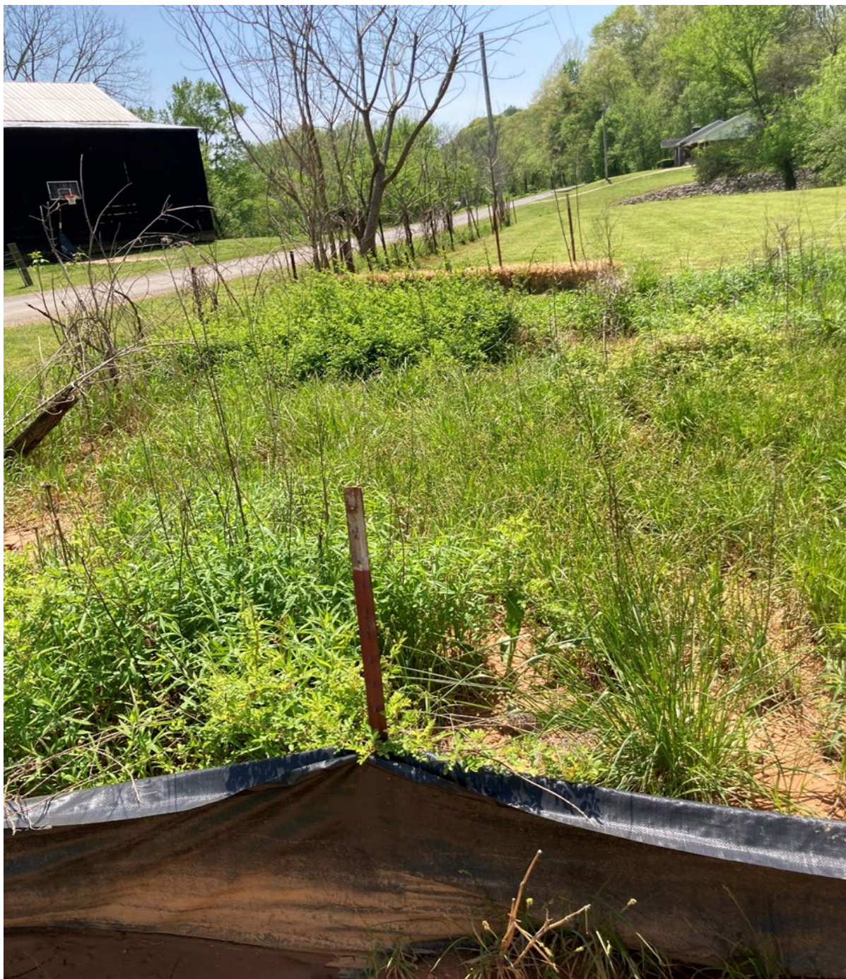
Photo 7: Series of BMPs at the facility entrance to treat stormwater before it leaves the site.
