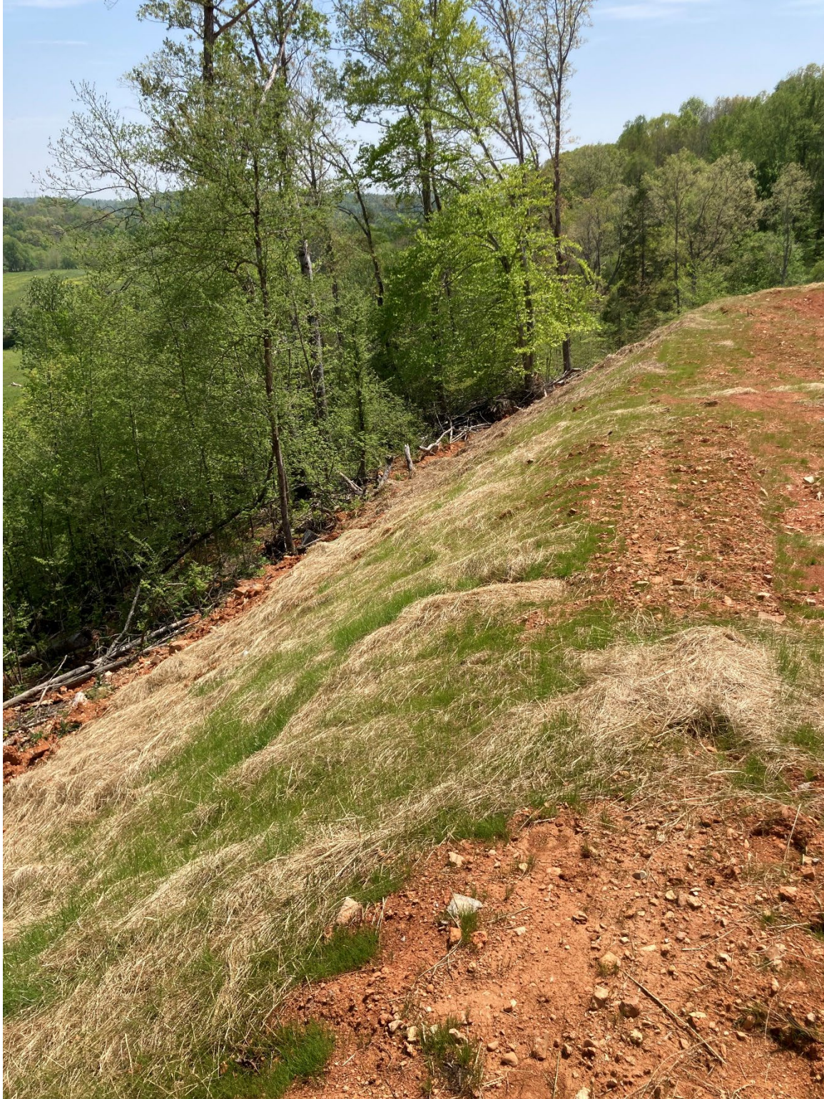
Photo 15: Photo of stabilized berm at the mine pit, note this berm could use more seed and straw.
