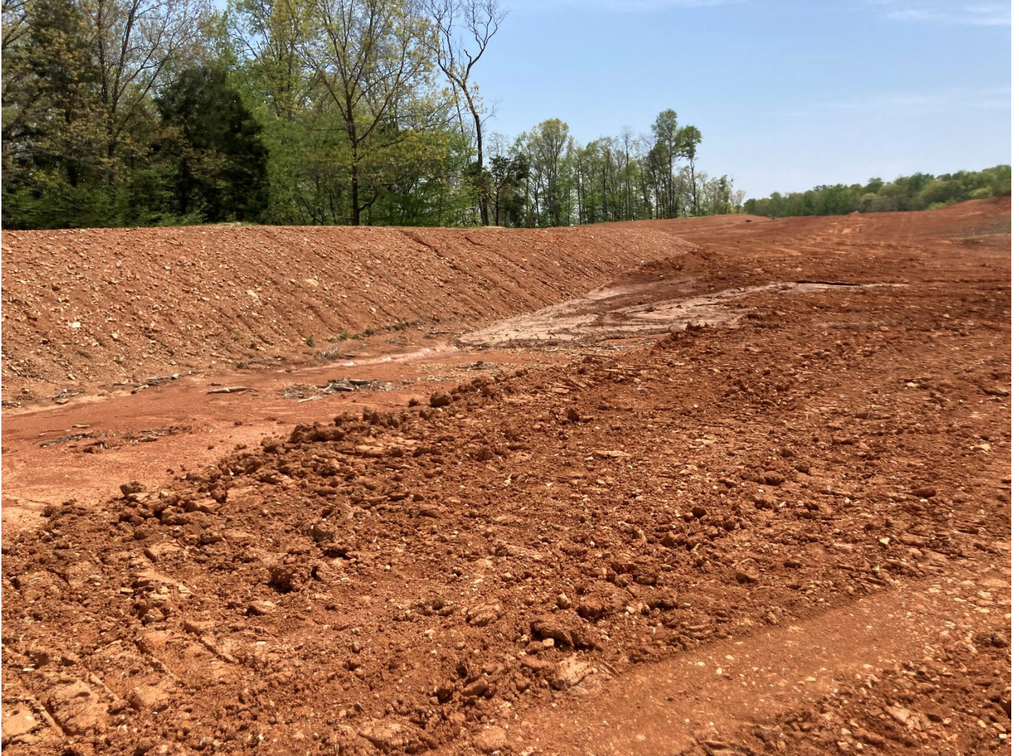
Photo 16: Large amount of disturbed area that does not drain to the mine pit or sediment basin. This area needs to be regraded to drain to the pit or treatment basin or be seeded or rocked if the facility does not plan to expand to this area soon.
