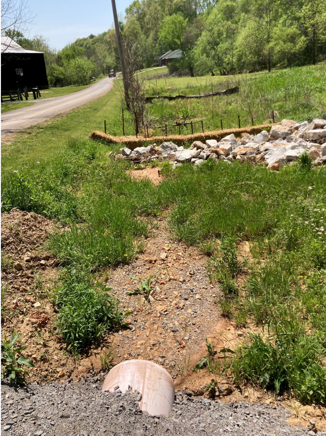
Photo 5: Road ditch culvert at the facility entrance and a series of BMPs below the culvert.
