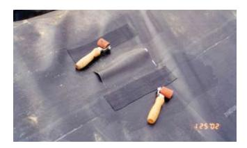
Any observed damage should be repaired immediately. Burrowing rodents that could damage the liner should be removed from the area.
