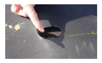
Figure 10E–29 Covered liner vent
