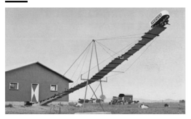
Powered thrower, or slinger, waste stacking equipment was once made for piling semi-solid waste conveyed onto it via a gutter cleaner. The power requirements were relatively high, and winds affected pile placement and development. Appearance and frozen waste buildup with regularly top-piled waste were also problems.
