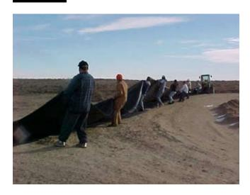
subgrade. To reduce stress on the liner, the trench should be backfilled during the cooler part of the day. The liner should extend down the side and across the bottom of the anchor trench. The corners of the anchor trench should be rounded, rather than squared, to reduce concentration of stresses at the corner.
