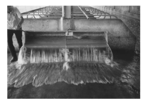
Air leakage and foreign material that restricts flushwater flow are siphon operation problems. Siphon flush tanks can be purchased, or they can be constructed from plans (MWPS 1976). Appendix 12A shows USDA Plan 6349 for a gutter flush system. Although vulnerable to puncture or cracking, molded glass fiber tanks are noncorrosive. Repair can be difficult. Stainless steel tanks are also noncorrosive, but generally more costly.
