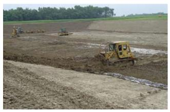
many compacted liners in ponds constructed using this method use 4H:1V slopes so that equipment will exert more normal pressure on the slope than downslope pressure.
