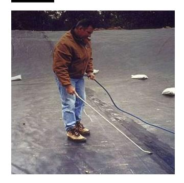
Figure 10E–18 Air channel test
