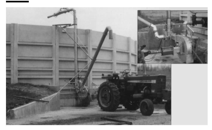
unless one or more impeller-agitators are mounted on the inside wall of the storage (see fig. 12–47). In most cases provision is made for adding dilution water near agitators for mixing of semi-solid waste. After agitation the pumpout valve is switched from agitation, and the pump is used to fill a nearby tanker spreader or to supply an irrigator for more liquid slurry.
