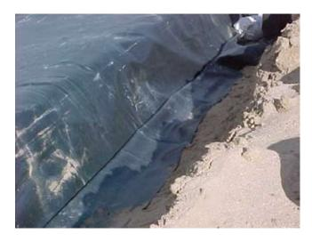
Figure 10E–10 Floating liner into place
