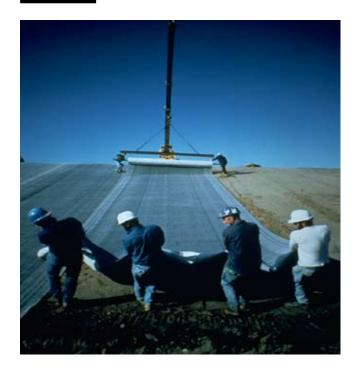
Figure 10E–6 Seams up and down the slope
