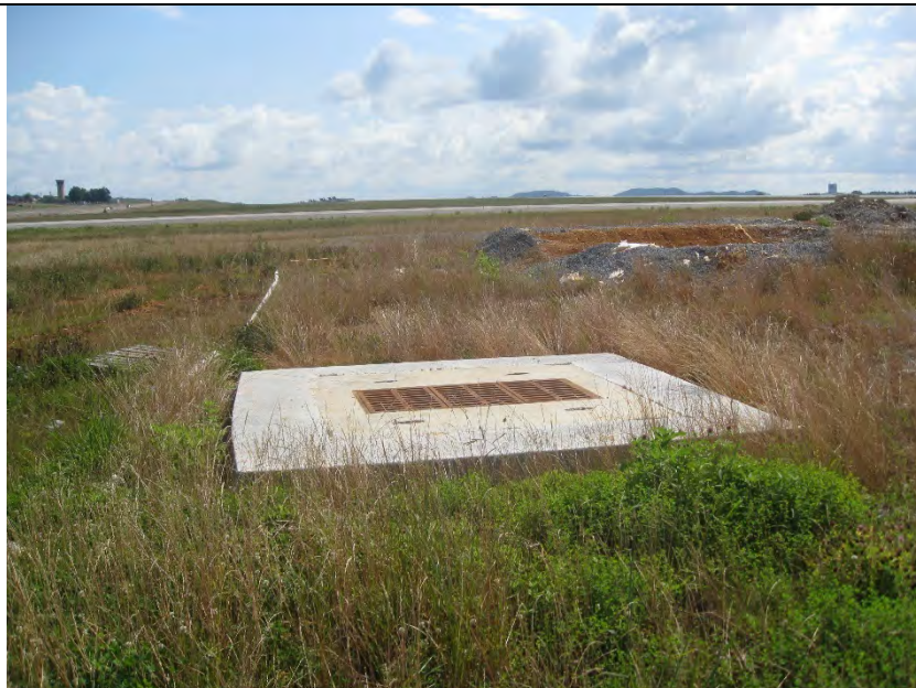
Photo 17 Concrete washout area Project 3
