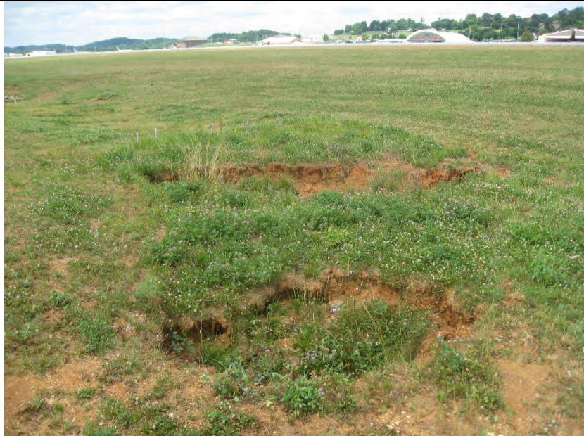
Construction fallout on Storm Line 2 between structures 204 and 206. Recommend coordinating remediation with CHA.
