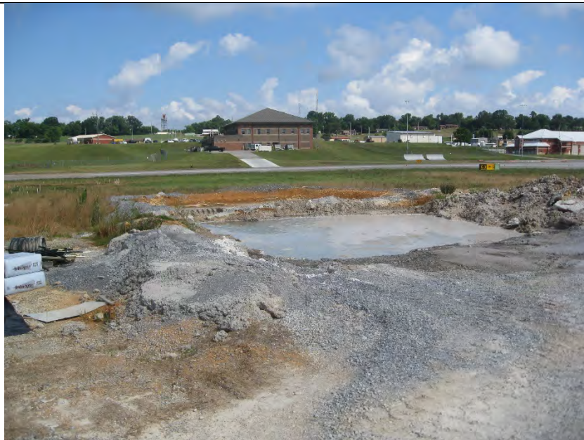
Photo 17 Concrete washout area Project 3
