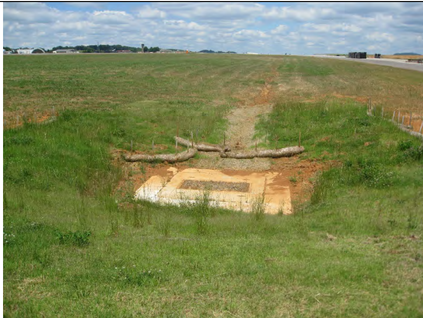
Structure 218. Erosion control blanket recently added. Recommend stabilizing bare areas. Recommend removing sediment from top of structure.
