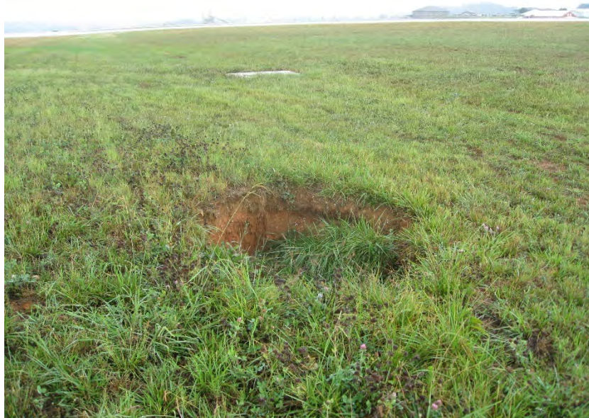
Construction fallout on Storm Line 2 between structures 206 and 208. Recommend coordinating remediation with CHA.
