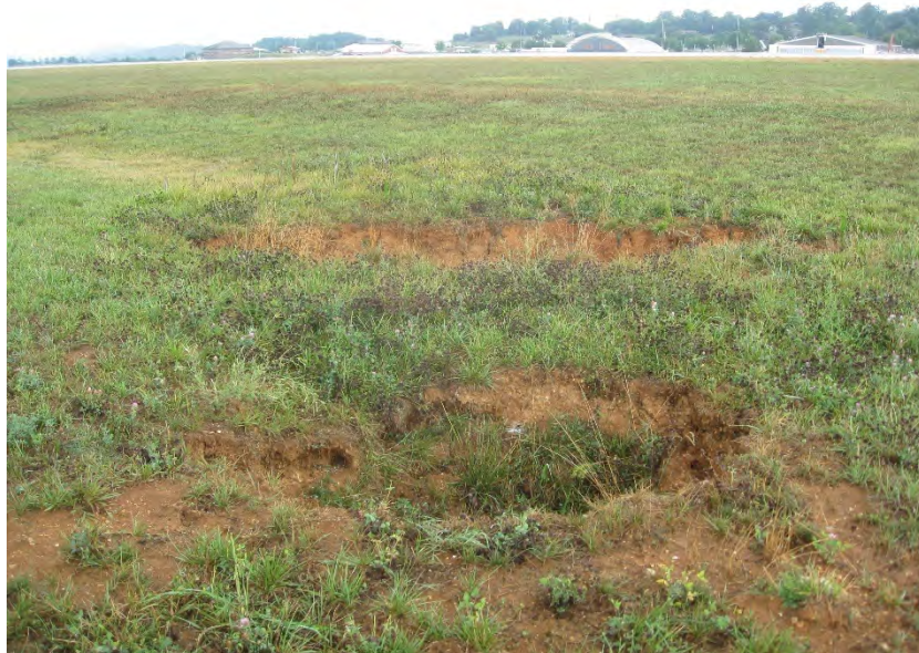
Construction fallout on Storm Line 2 between structures 204 and 206. Recommend coordinating remediation with CHA.
