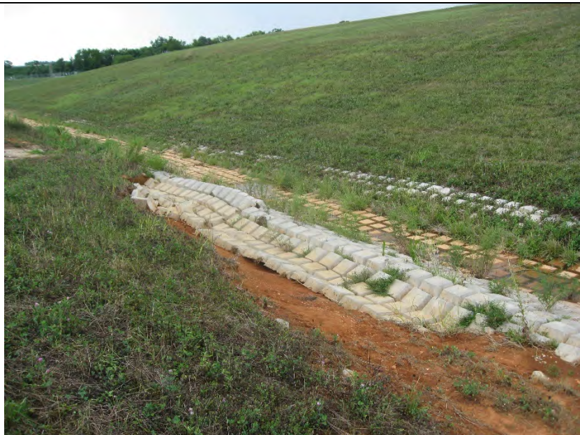
Below structure 224. Side slope has eroded causing damage to the articulated concrete block. CHA, Harper and KMAA were already aware of the issue as discussed in a progress meeting dated 07/16/2020.
