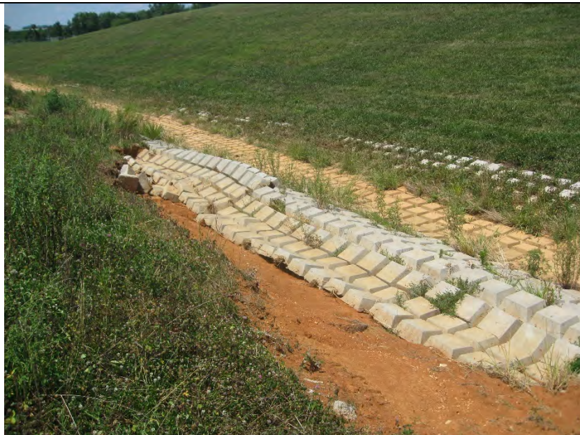
Below structure 224. Side slope has severely eroded. CHA, Harper and KMAA were already aware of the issue as discussed in a progress meeting dated 07/16/2020.
