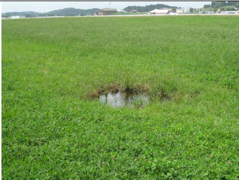
Potential construction fallout on Storm Line 2 between structures 204 and 206 just downgradient of an underdrain outlet. Recommend coordinating remediation with CHA.
