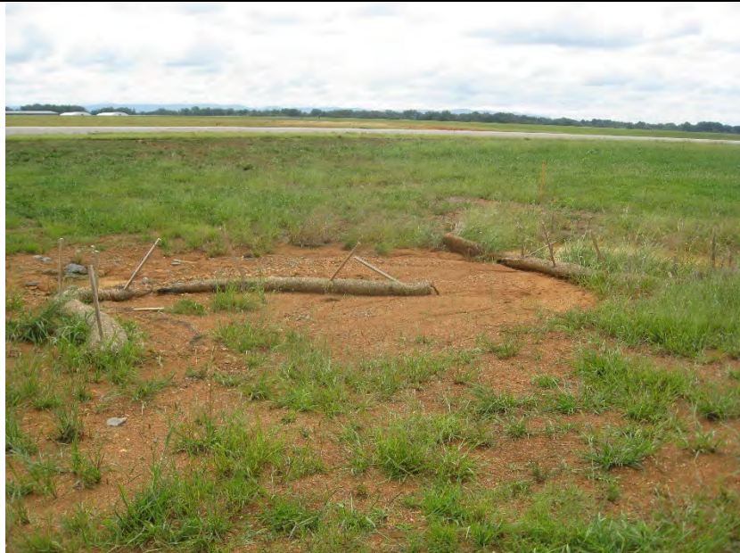
Structure 212. Recommend repairing eroded ditch line Recommend removing sediment. Recommend replacing all sediment tubes. Recommend stabilizing remaining bare areas.
