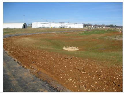
Entry Code: S Action Code: Above existing structure #120. Edge of pavement recently saw cut in preparation for backfill operations.
